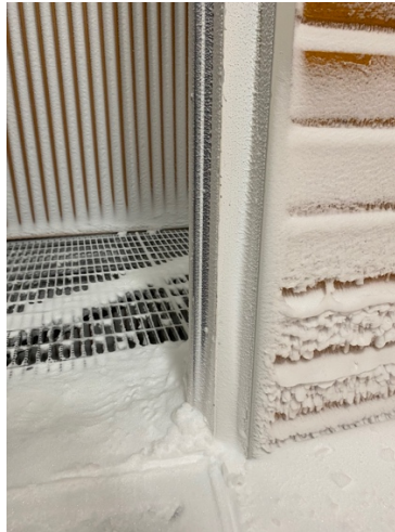
Snow building up in my door frame, causing the door to jam
