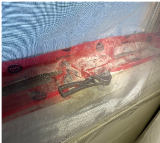
A window that has been covered to keep heat from escaping
